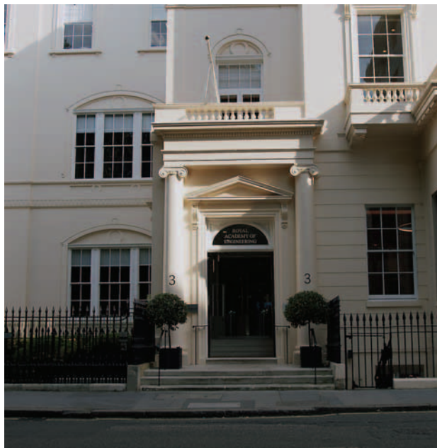
Above, Royal Academy of Engineering, Prince Philip House, 3 Carlton House Terrace, London
